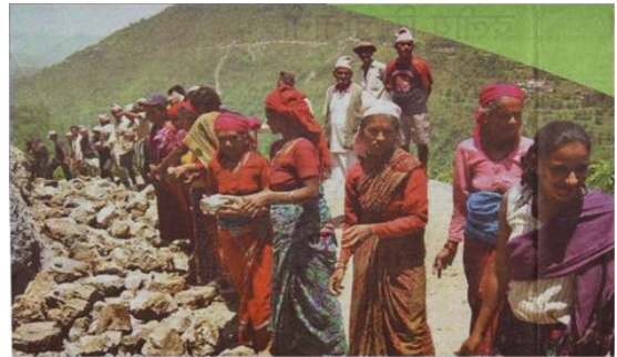
Stakeholders collaborating on project (Source: SDC)
